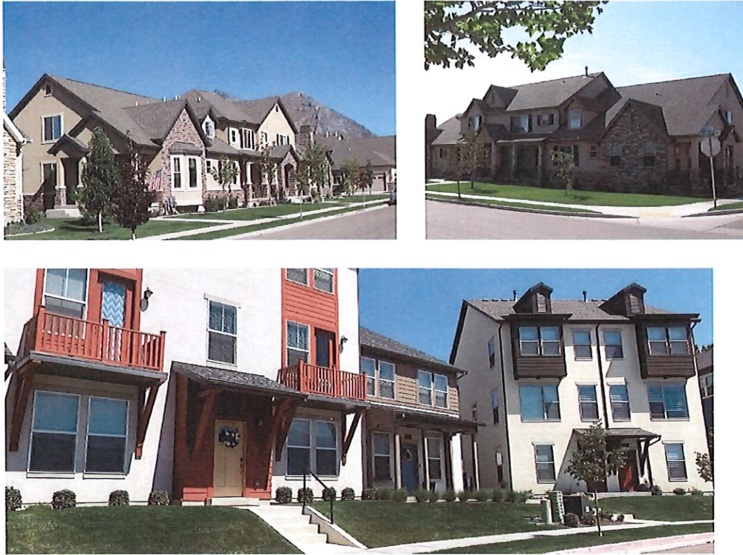
Figure 7. Twin home Examples: Pictures are representative examples. These homes face the street and have rear loaded garages.
